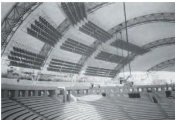
Figure 9 – Interior view showing the sound absorptive panels at the rear zone of the amphitheatre
