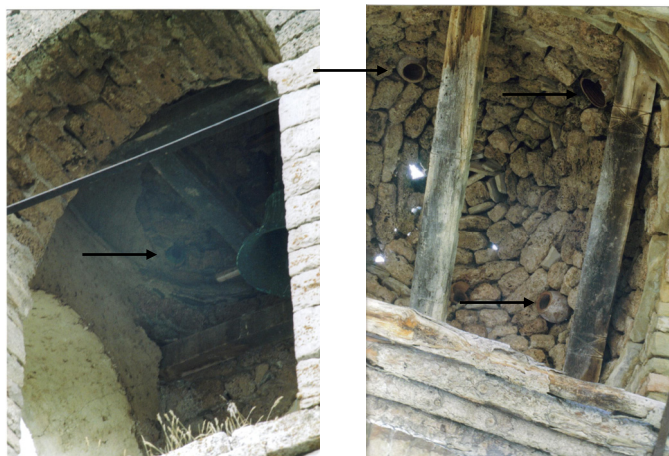
Figure 7 – Pottery located in church towers (arrows)
