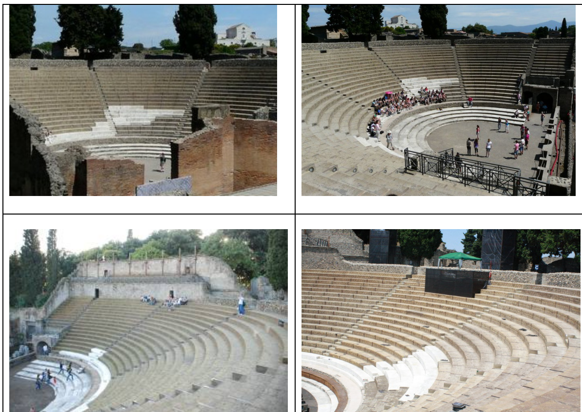
Figure 4 – The “Large Theatre” in 2011, after restructuring works
