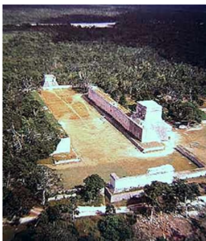
Fig 6 - Recent photo of Great Ball Court. Notice the two end temples are located on the center line and are not in physical contact with the two long parallel walls of the playing field. The walls are 28 ft. tall and 278 ft. long, precisely parallel, and highly sound reflective.
